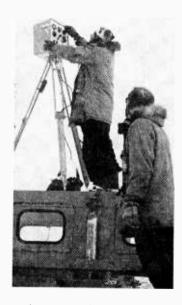
Distances across the vast and eerie Antarctic wastes were measured using electronic survey equipment. Protected by warm parka and beard, Boeing man adjusts the equipment which was mounted on snow vehicle to get it above the snow-whipped ground surface. As shown at the top, the men relaxed by conquering a mountain of snow near camp.
