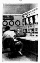
Television receiver screen on console is one of three that monitors activity in the three rooms or chambers of oxygen tank facility. Here, as in any form of technical communication, a picture is worth a thousand words, or in this case, it is worth valuable time that might be as in diagnosing meter readings when a picture might reveal the nature of the situation within the oxygen chamber
