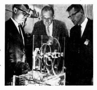
Boeing Company antenna experts T. L. Johnson, Robert Tighe, and Arthur Guy study the electrical impulse generator they designed for subsurface antenna experiments in the Antarctic. One of the Boeing team, shown below, has his turn at the morning chore—digging antenna cable and supplies out of snowbanks constantly formed by drifting snow.
